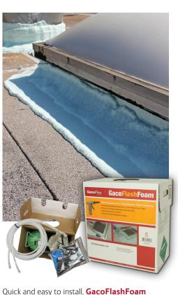
Spray-Applied 3 lb. Polyurethane Foam Flashing provides an economical and superior alternative to labor intensive seam tapes. The convenient self-contained kit is designed for use as spray-applied flashings at curbs, parapets, walls and penetrations prior to application of GacoFlex Coatings.
