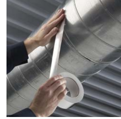
Sealing duct work
