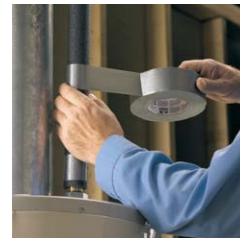
Installing and repairing
