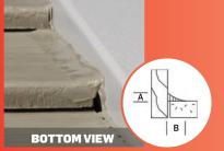
• Dimension A under ¼" minimum. This will compromise the sealants adhesion performance and ability to sustain joint movement capability • Reduced sealant volume will diminish sealants ability to accommodate joint movement
