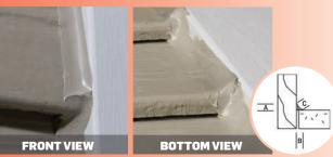
Dimension A and B are covered by a thin layer of sealant. Overtooling reduced sealant volume necessary to accommodate joint movement
