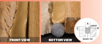
• Dimension A and C meet the required standard but overtooling reduced sealant volume necessary to accommodate joint movement causing separation • Dimension B below standard depth (shallow depth of this sealant will not provide optimum performance). Excessive sealant removed due to overtooling.
