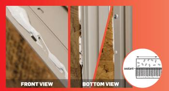
Substrate movement will smear the sealant breaking down the capacity to maintain a gasket seal. This will leave insufficient amount of sealant to accommodate joint movement allowing for air and moisture infiltration
