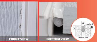
Dimension C beyond standard maximum depth. This will debilitate joint movement capability causing fissures and fractures
